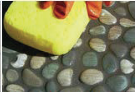
Repeat sponging off the grout until the desired look is reached. Look for narrow grout lines between pebbles. Once the grout has completely dried seal the tiles a final time.
