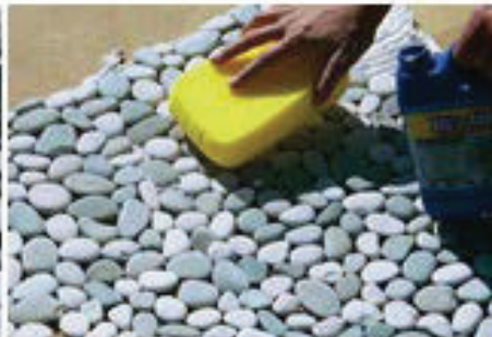
Seal the tile with a good quality penetrating sealer. Color and shine enhancers can also be applied to vary the finish off the pebbles.
