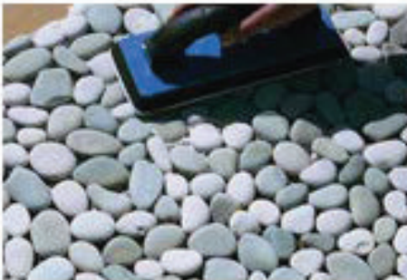
Lightly tap down the tile without pushing the pebble into the thinset.
