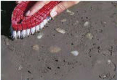
When grout has dried for 30 minutes use a stiff bristled brush to remove the excess grout.
