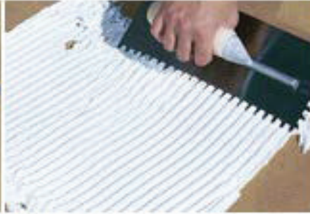
Apply thinset with a trowel.
